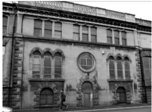
The central section of the Newark Works, which would be just as at home on the Grand Canal in Venice
