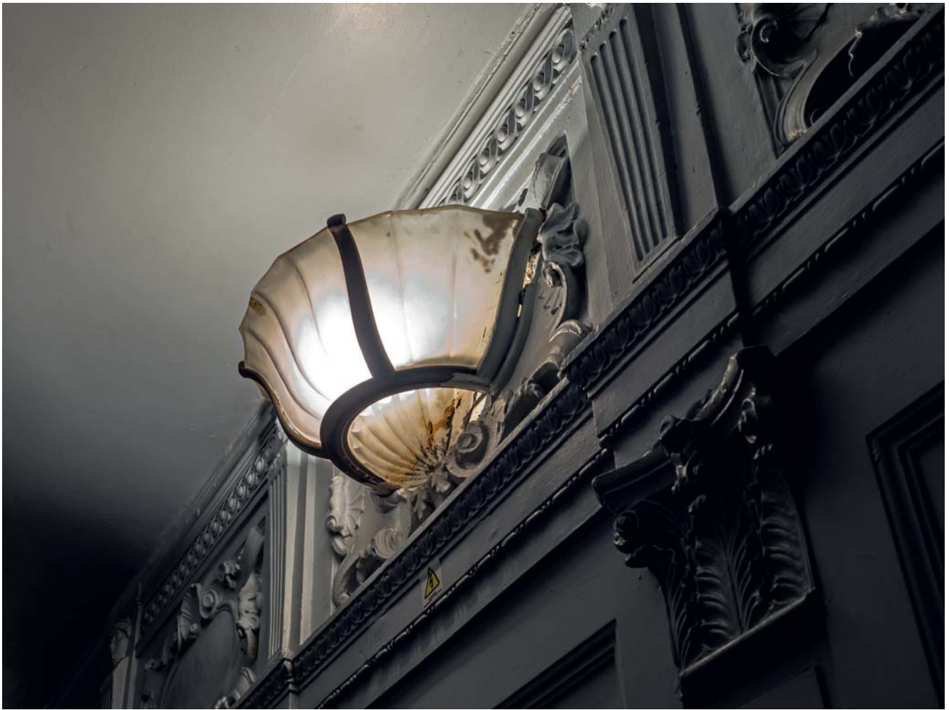
The original 1920s decoration with wall panels and light fittings is still visible in many places (image: Ian Grundy).
