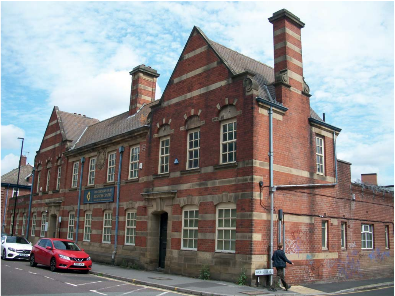
Former Coroner's Court, Sheffield (image: Cllr Douglas Johnson)
