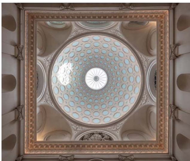
In the Great Hall (left) the carpets have been removed, the original stone floors exposed and repaired, and most spectacularly, the 1780s glass screen uncovered and reinstated. Following paint scrape analysis throughout the building the Great Hall and its dome (above) has been redecorated in the original colour scheme (image: Emli Bendixen).
