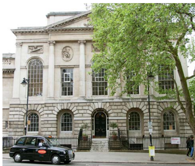
The fine main façade of the Sessions House overlooks Clerkenwell Green. The stone and render of the external elevations have been carefully cleaned and renovated, reopening original windows, reinstating railings and gas lights (image: Emli Bendixen).
