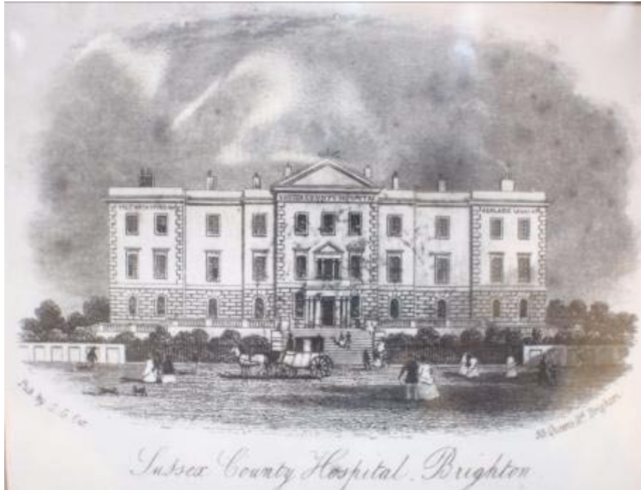
Hospital with Victoria and Adelaide wings c.1841 (Brighton History Centre)
