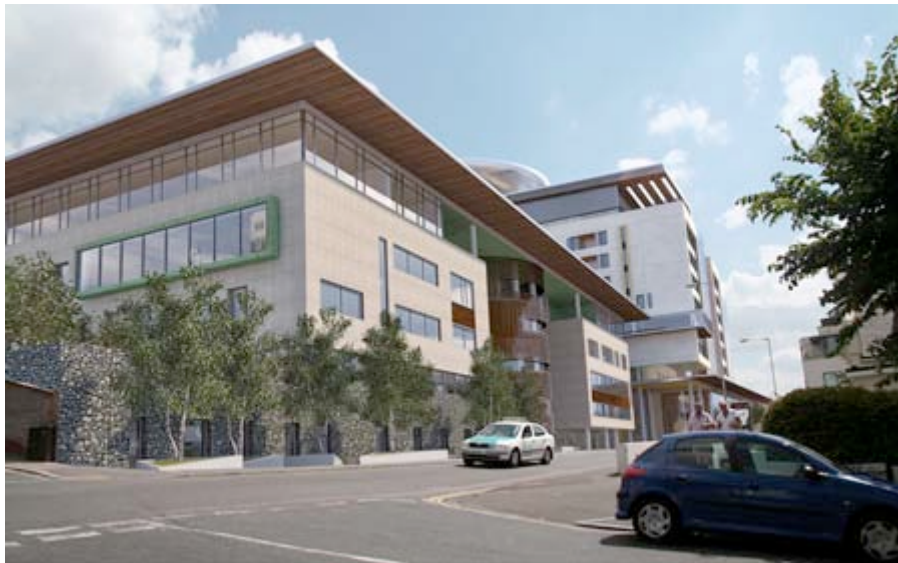
The proposed replacement block seen from the west, along Eastern Road
