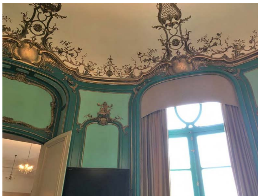
Plasterwork, Bar Lounge, Esher Place
