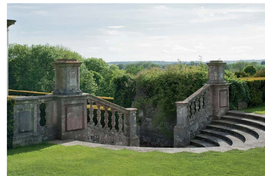
Circular steps, Marshcourt, Hampshire (registered Grade II*)
