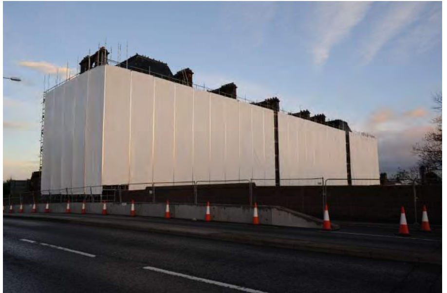
The station hotel under scaffolding, autumn 2018
