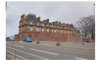
VIEW FROM SOUTH WEST
