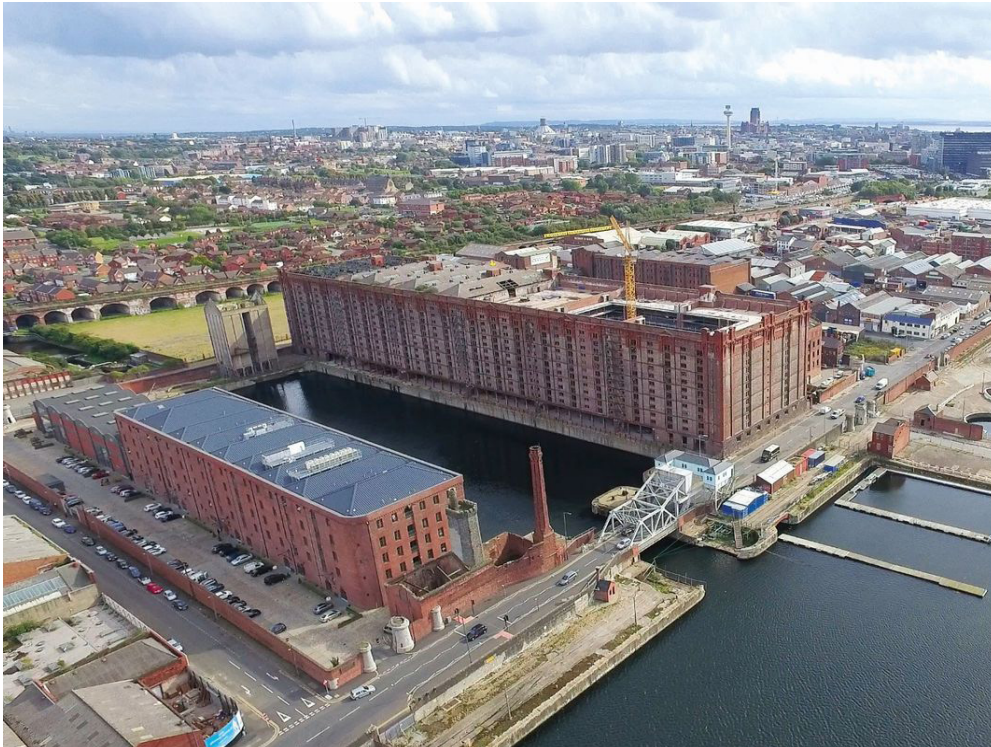
Aerial view of the Tobacco Warehouse overlooking Stanley Dock (Credit: Tobacco Warehouse)
