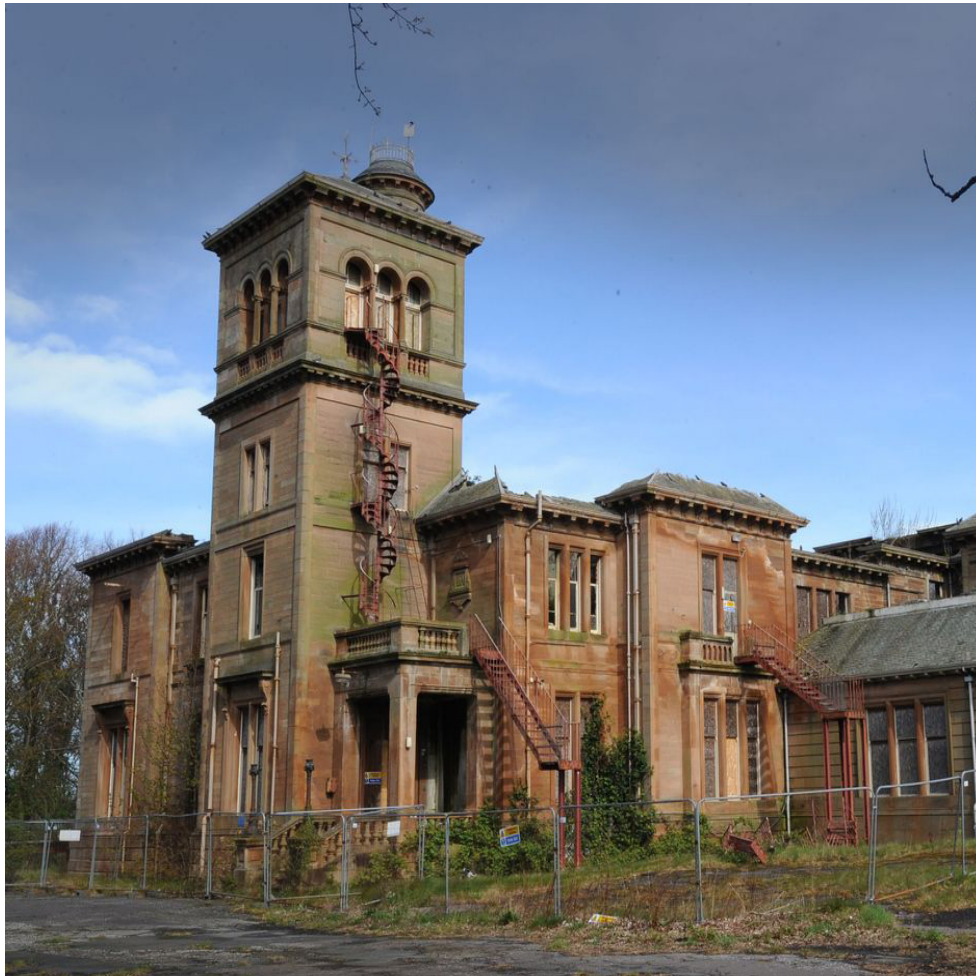
Seafield House following the fire in 2008 (Credit: Alamy)
