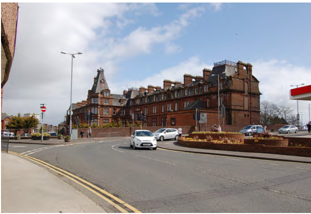
VIEW FROM WEST
