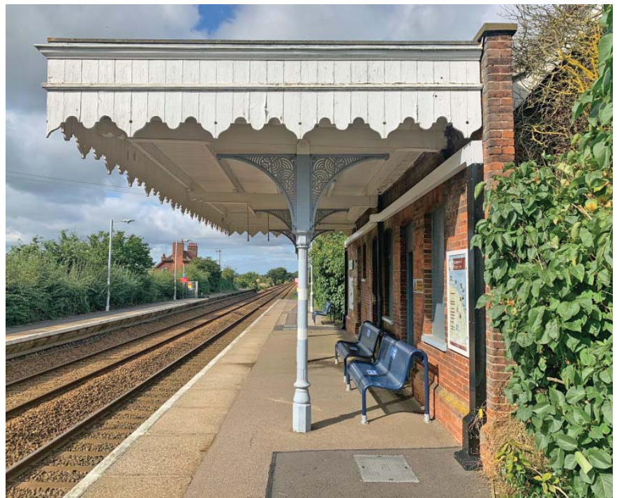
The cast iron columns beneath the canopy at Salhouse have decorative oriental patterns (Credit: Gerard Stamp)
