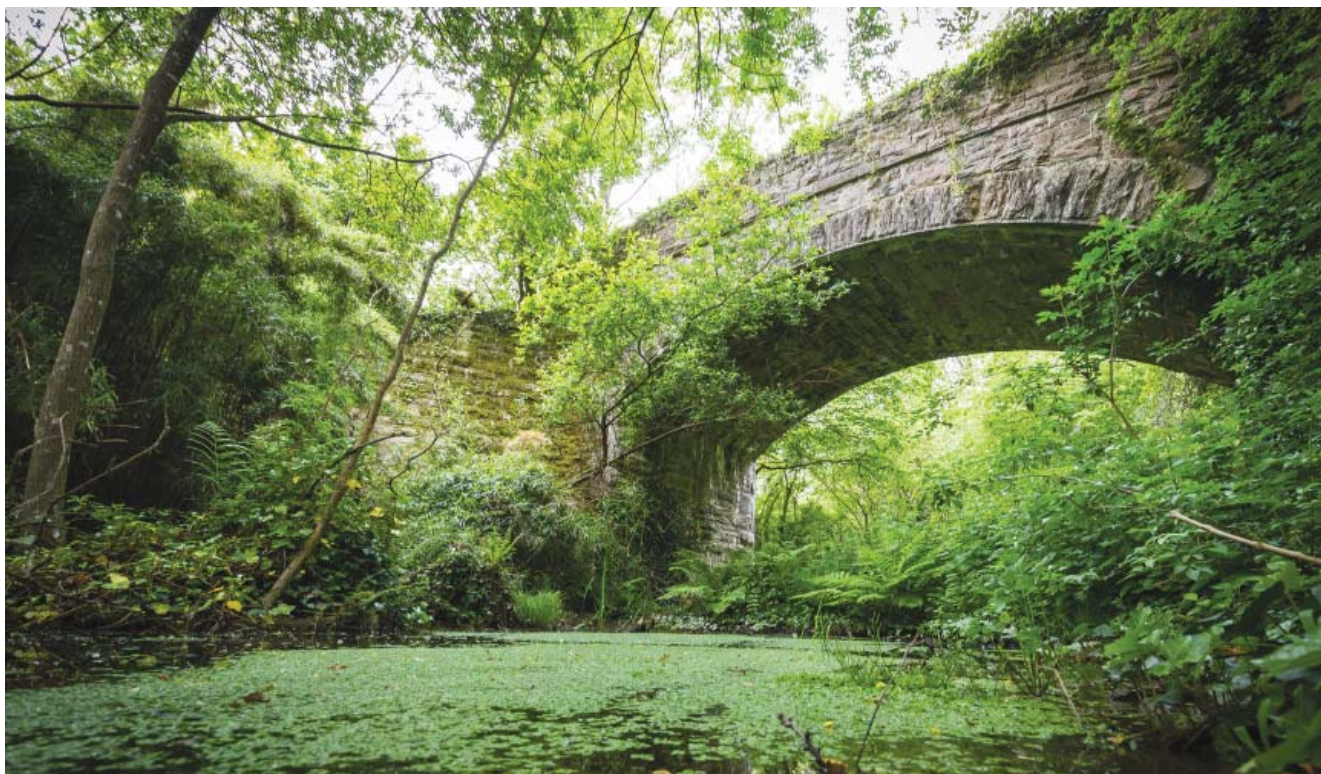
Isambard Kingdom Brunel designed this bridge near Saltash which National Highways intended to infill (Credit: The HRE Group)
