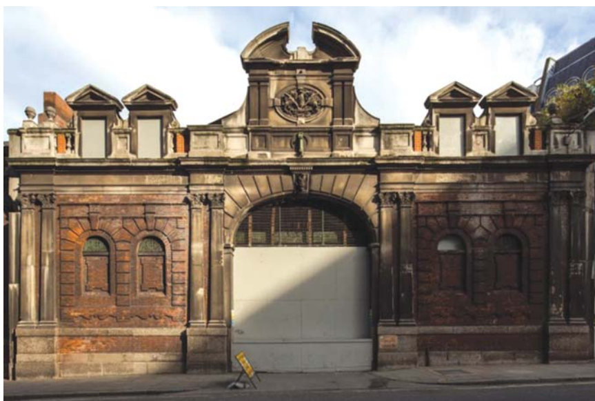
The former Smithfield Fish Market building on Snow Hill (Credit: SBH)
